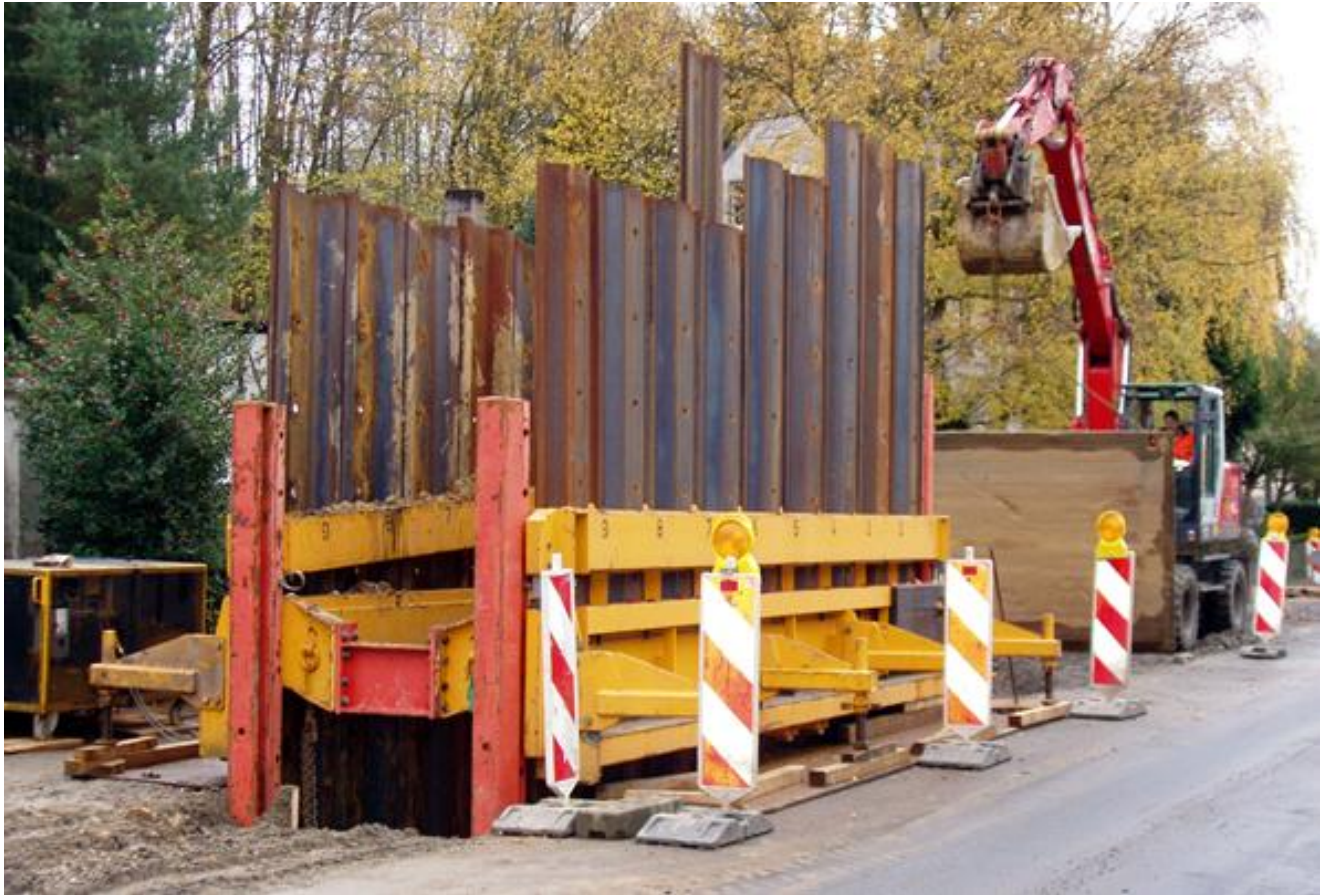
↑ Sheet pile machine DPV
