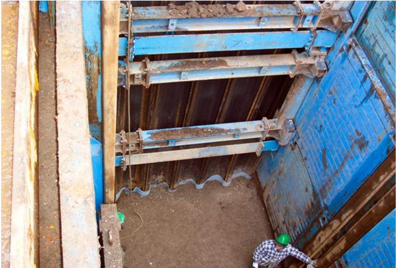
↑ Head shoring with sheet piles
